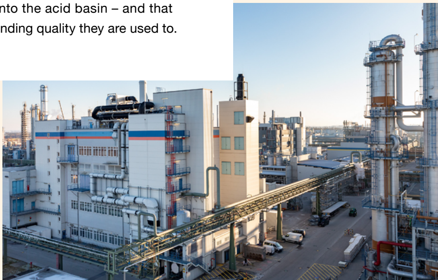
The existing polysilicon-cleaning building in Burghausen. WACKER is currently building another cleaning line at a cost of around €300 million, which will increase cleaning capacity for semiconductor-grade polysilicon by well over 50 percent.
